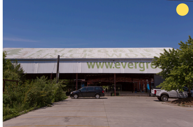
South Pavilion Entrance 2
